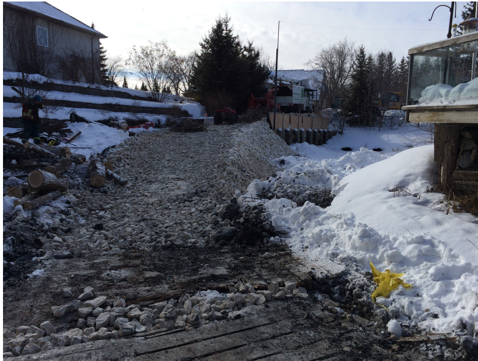
Photo 2 - Temporary site access ramp at Tartan Way culvert.
