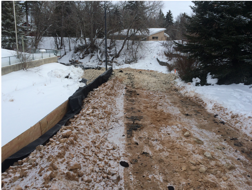
Photo 1 - Temporary site access ramp at Tartan Way culvert.
