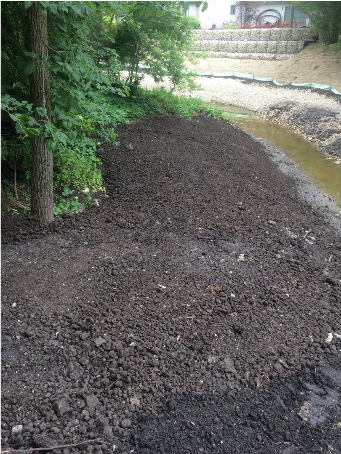
Photo 3 - Topsoil placed on rockfill toe and area required to remediate at 3154 Henderson Highway.
