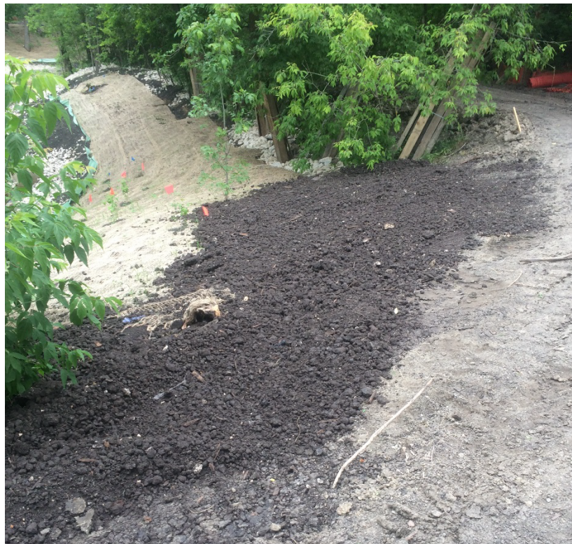
Photo 1 - Topsoil placed on rockfill toe berm at 3144 Henderson Highway.
