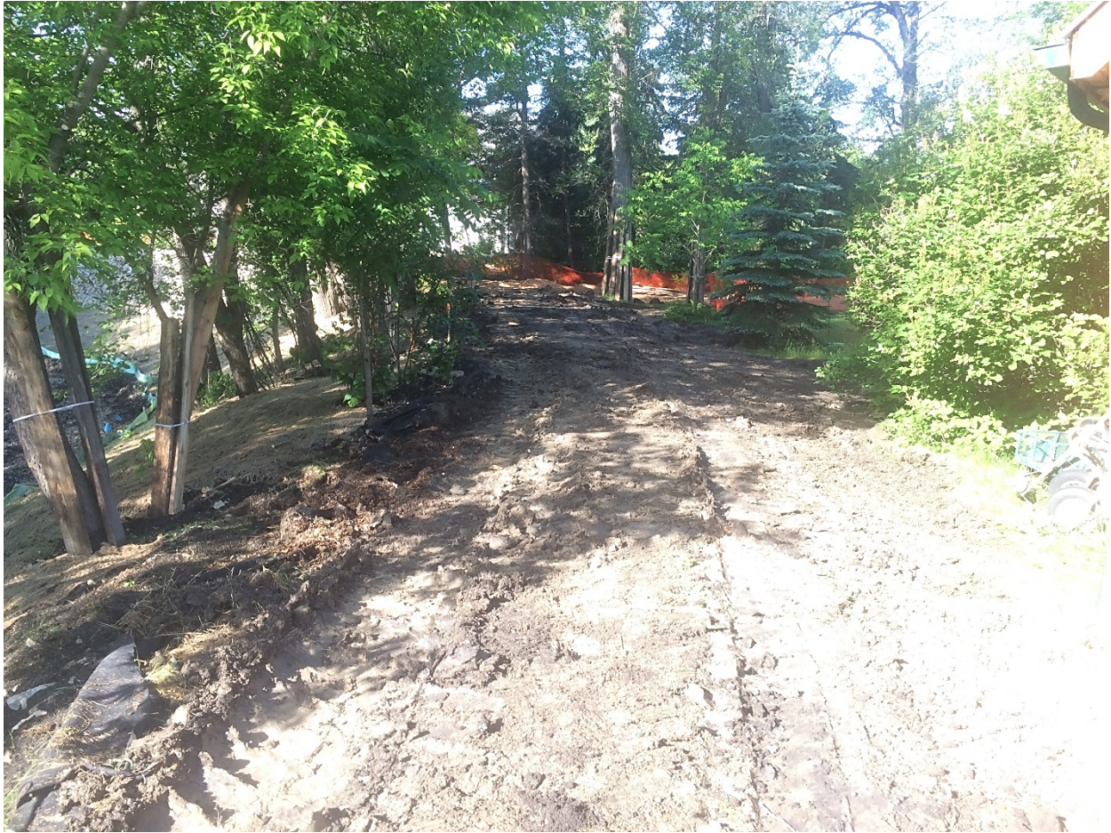
Photo 9 - Organic material removed from existing dike at 1040 Highland Park Drive.
