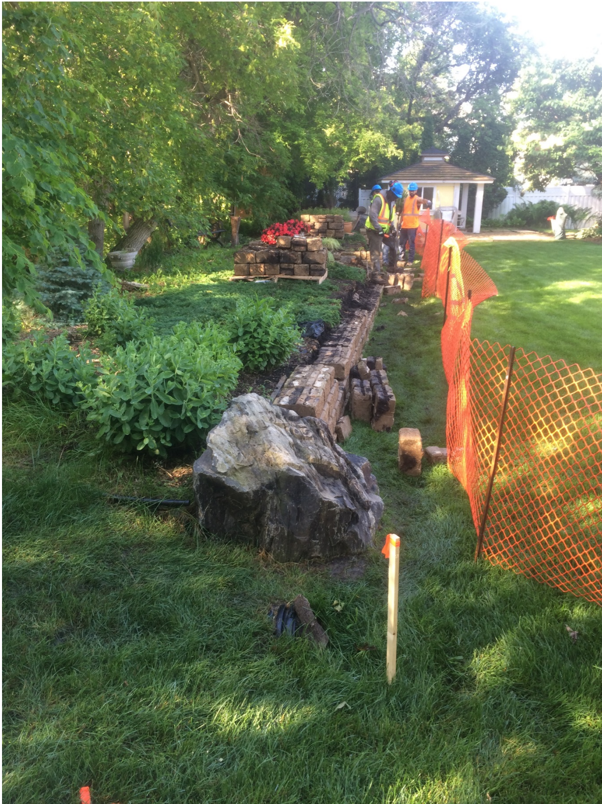
Photo 11 - Removal of the existing segmental block wall at 1020 Highland Park Drive.
