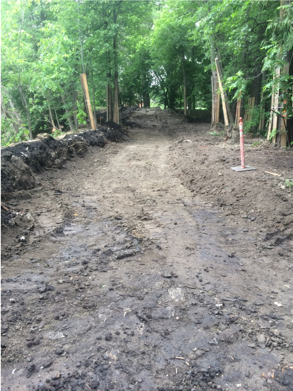
Photo 4 - Existing dike and organic material below existing dike removed at 3154 Henderson Highway.
