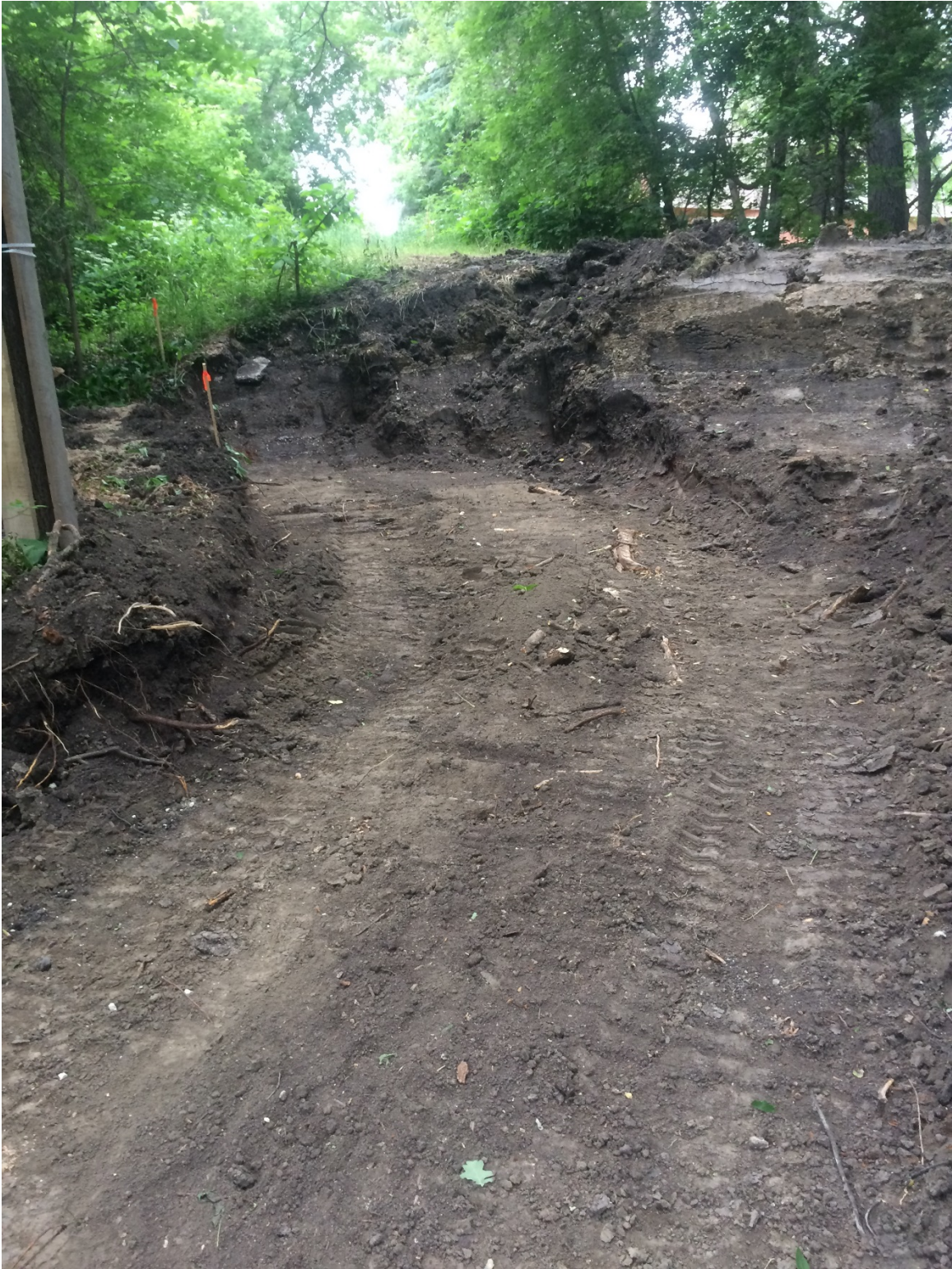
Photo 5 - Existing dike and organic material below existing dike removed at 3154 Henderson Highway.
