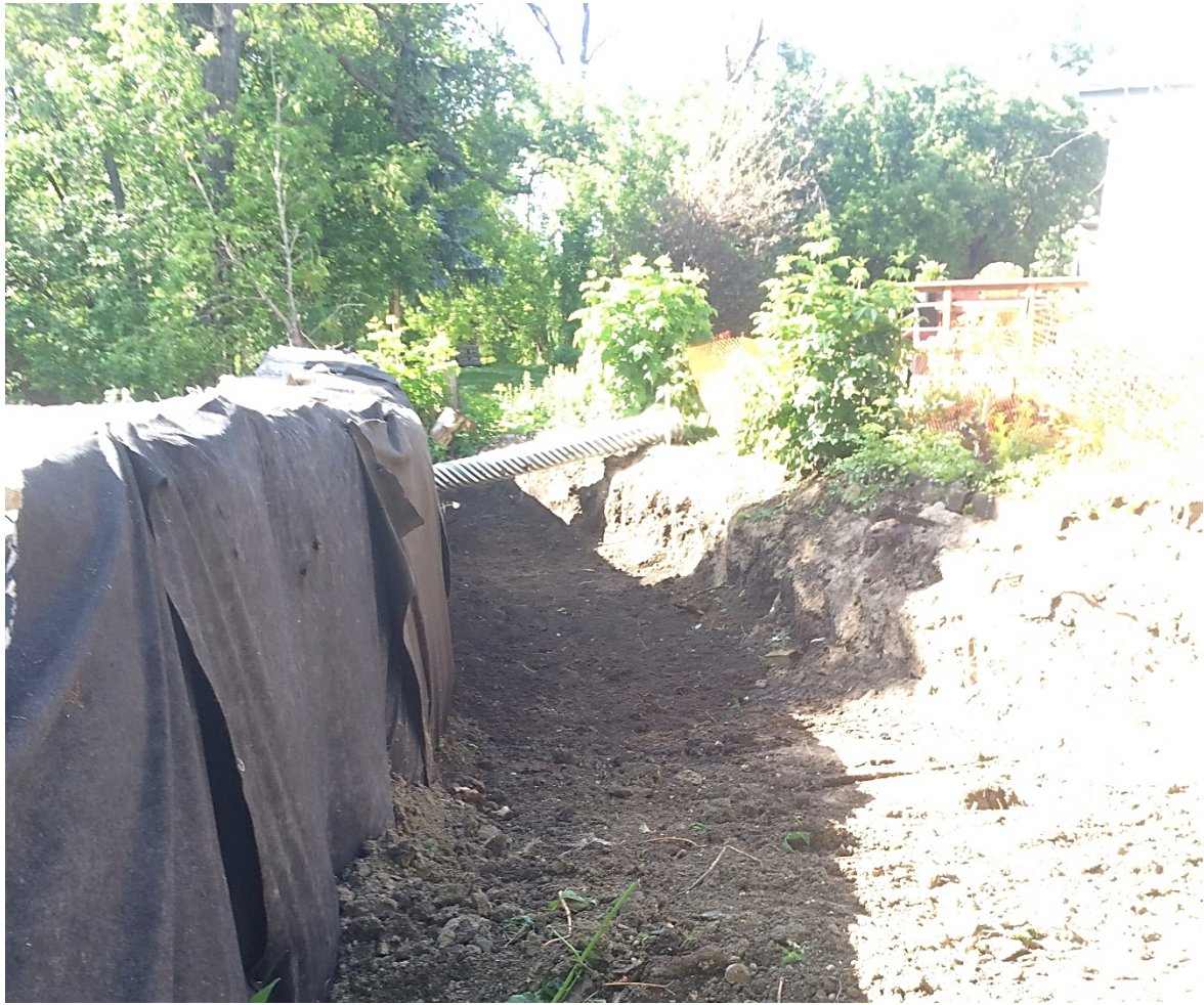
Photo 10 - Organic material removed and clay fill placed behind gabion baskets at 1030 Highland Park Drive.
