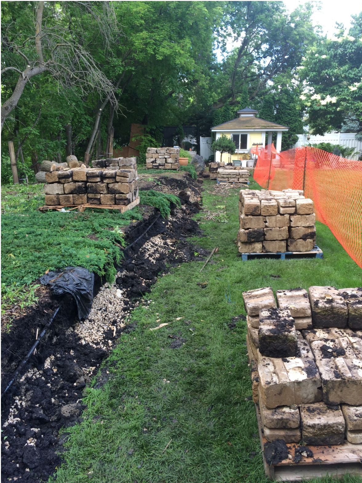
Photo 12 - Removal of the existing segmental block wall at 1020 Highland Park Drive.
