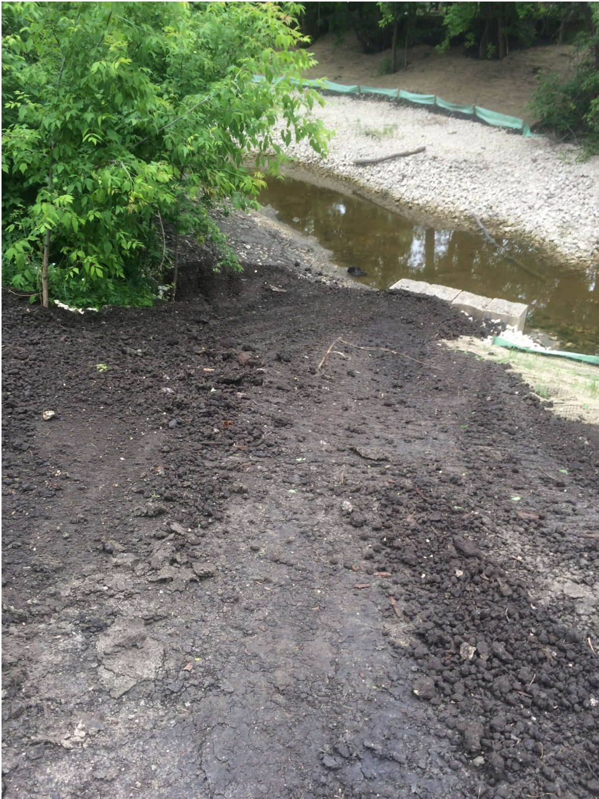
Photo 2 - Topsoil placed on rockfill toe berm at 3144 Henderson Highway.
